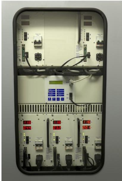
Fig 4. Typical Line-Interactive UPS used in datacenter
